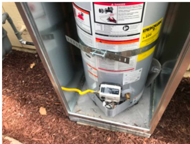
Unsafe Installation of Water Heater Gas Line
